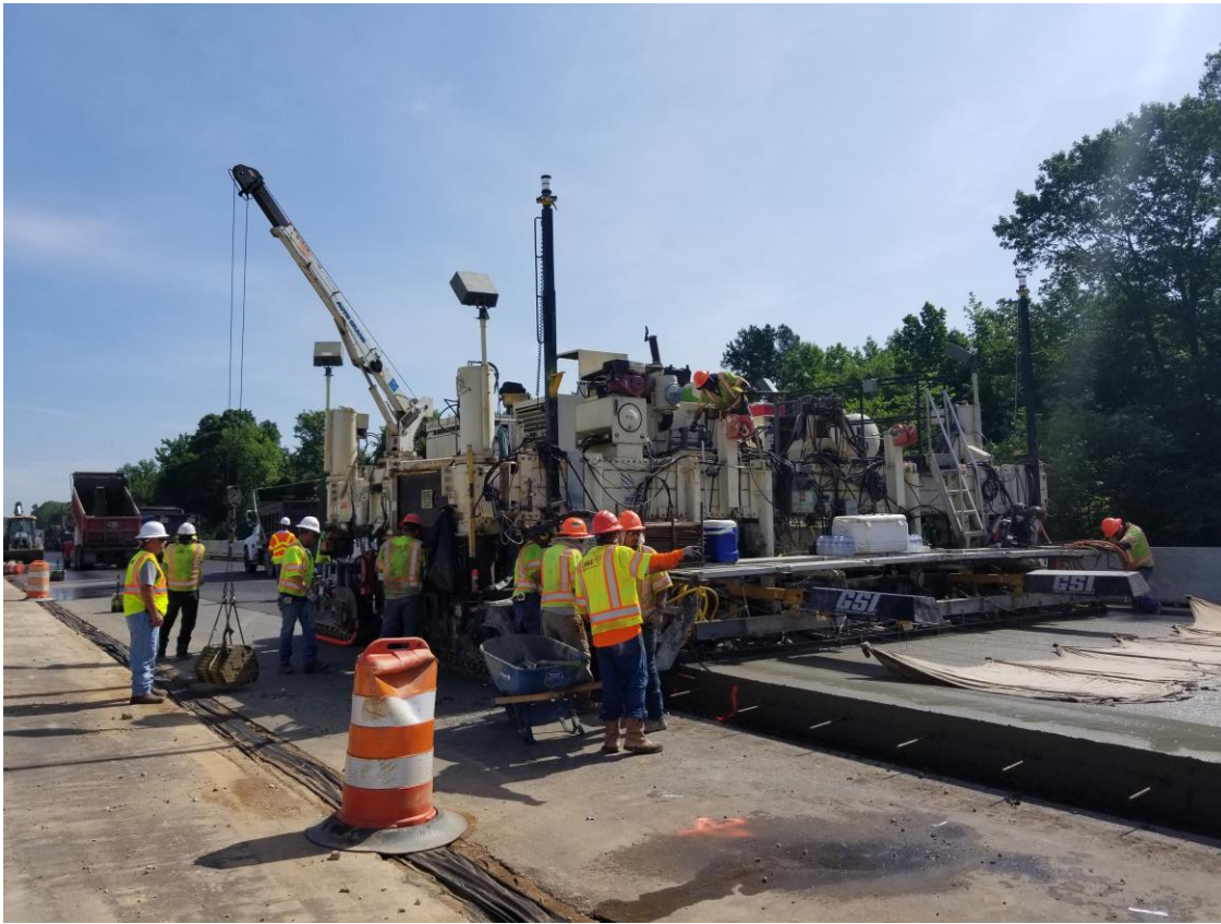
Figure 8: G&Z paver with 24 foot width, DBI technology, and Gomaco GSI real-time smoothness used for mainline pavement.
