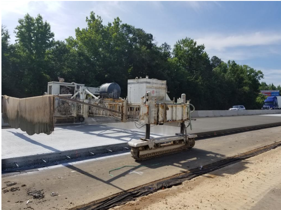
Figure 10: Application of curing compound.
